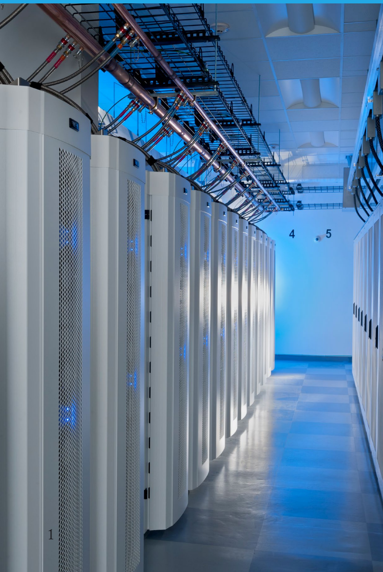
Internal rack space is not affected by the rear doors
